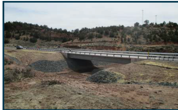
Location: Kinlicee, AZ Client: BIA Project: Cast-in-Place Bridge w/ Erosion Protection
