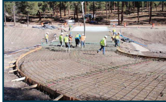
Location: Santa Clara, NM Client: Federal Highway Administration Project: Concrete Rigid Paving
